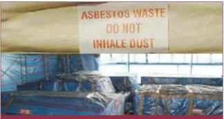
Removed asbestos sheets are properly wrapped with polyethylene sheets and labelled
